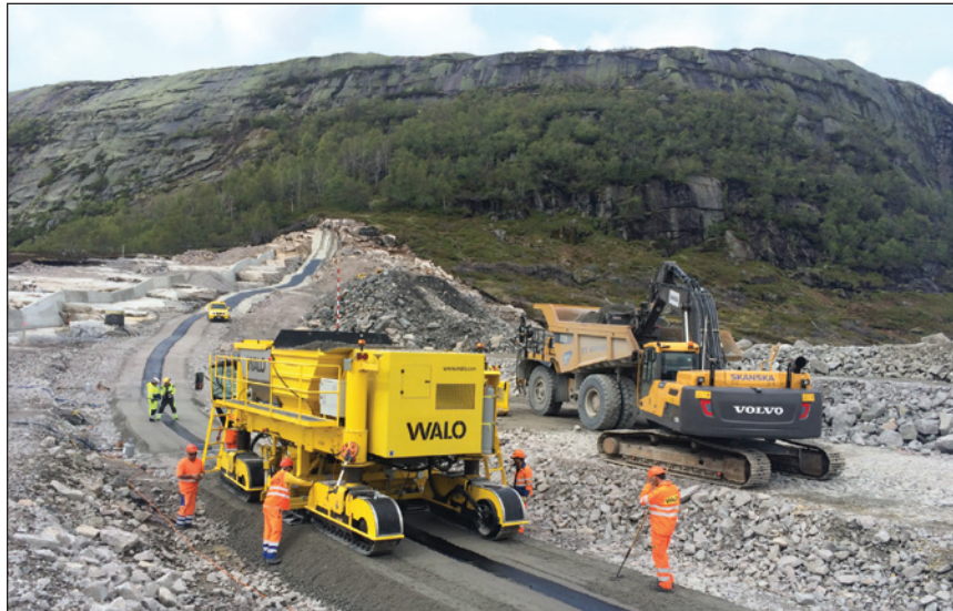
WALO installs an asphalt core in a dam in Norway.
