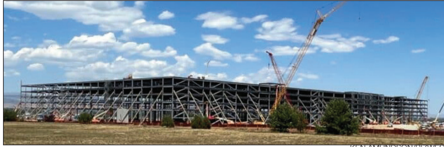
As of late July, the 3.8-million-square-foot Amazon center under construction in north-east Loveland was taking shape.
