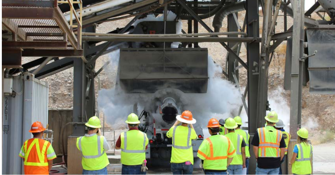
A batch plant uses the NITROcrete system of cooling the aggregate.
