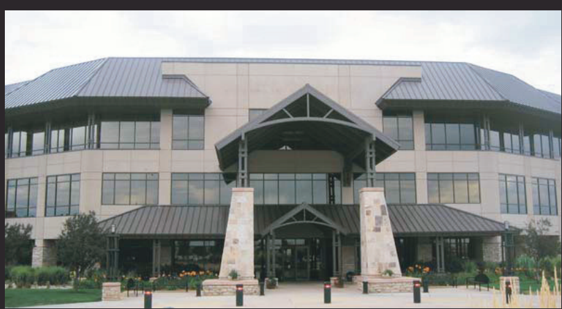
SWIFT AND COMPANY TORNADO REPAIR - GREELEY, COLORADO
