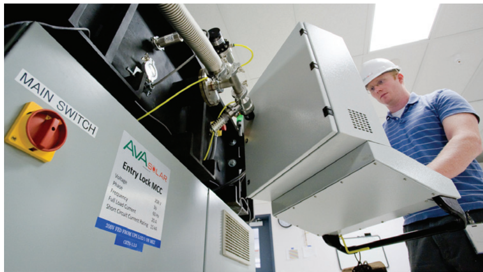
Courtesy Abound Solar
