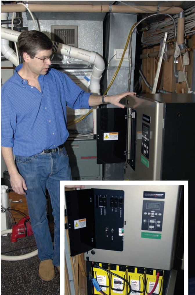
COURTESY ALISON PICHER Andrew McKenna installed "smart" technology in his Boulder home to help monitor his family's energy use. McKenna isn't hooked into Xcel Energy's Smart Grid, but has the capability to do so. His system also has a battery backup that can provide electricity to his home during a blackout.
