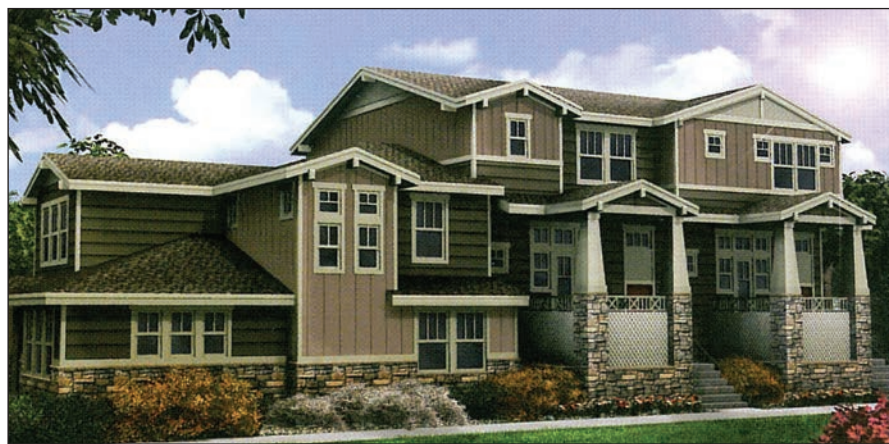
COURTESY BOULDER CREEK BUILDERS
