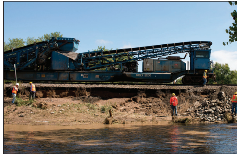
Workers repair a railroad crossing damaged by flood waters.
