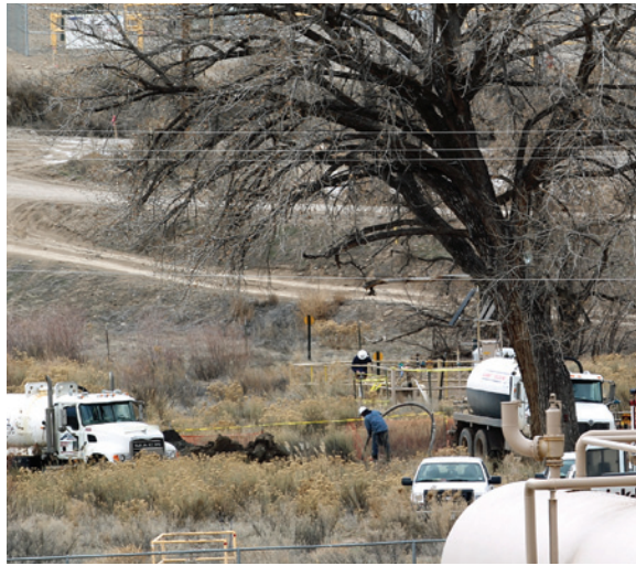
COURTESY DEAN HUMPHREY, GRAND JUNCTION SENTINEL Crews work to clean hydrocarbon spill near Parachute Creek.
