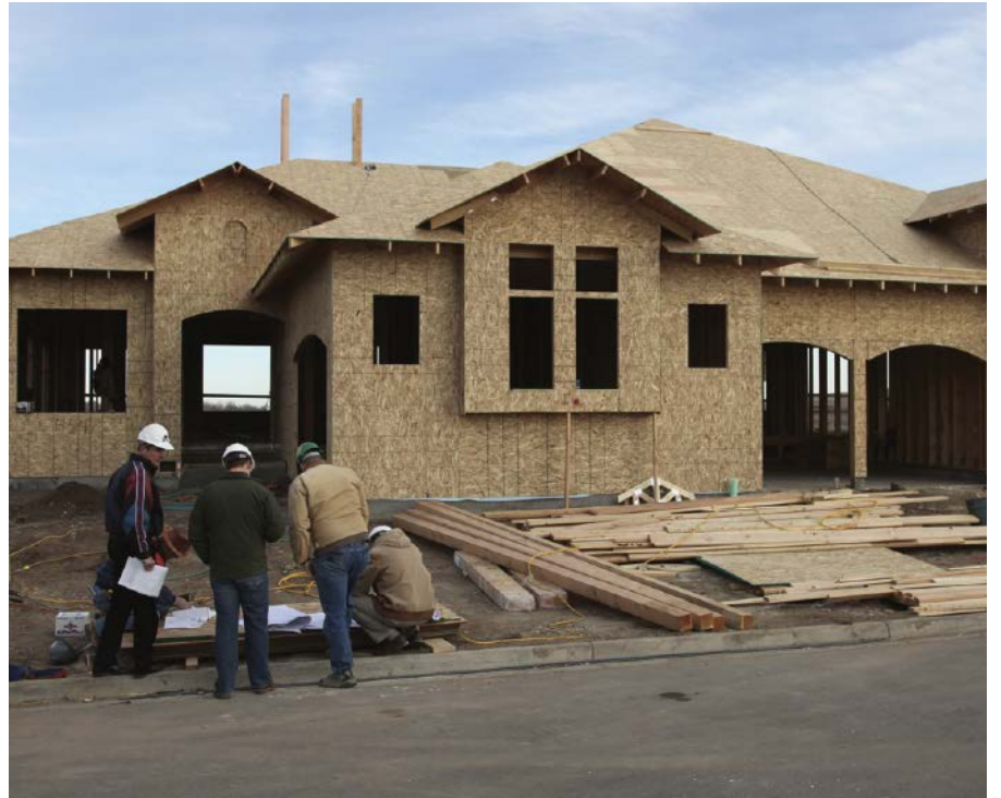
Courtesy Boulder Creek Builders
