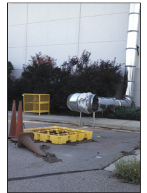
BUSINESS REPORT PHOTO Special vents hang off the abandoned Abound Solar plant in Longmont.
