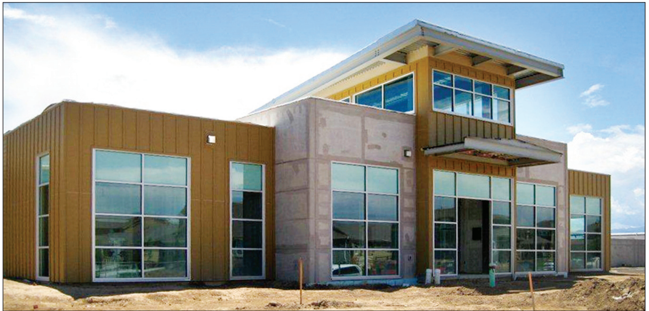
COURTESY PINKARD CONSTRUCTION CO.
