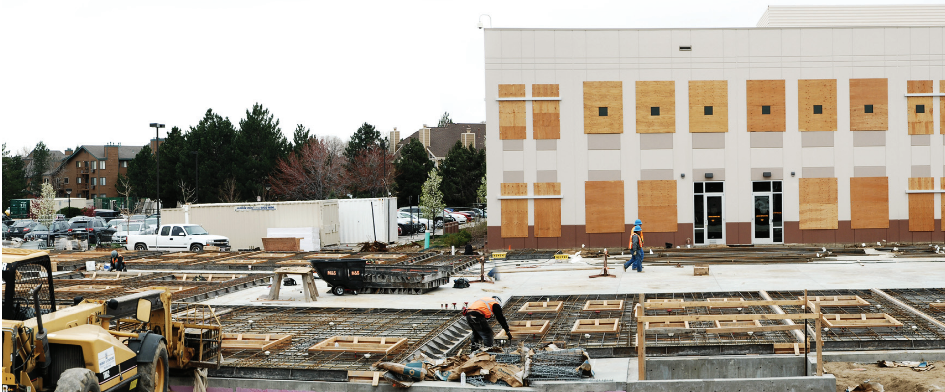
The foundation is nearing completion for Covidien Plc's 63,000-square-foot Innovation Center at the medical-device maker's campus in the Gunbarrel neighborhood of Boulder. It is expected to be open
