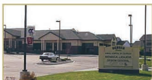
1721 W Harmony, Fort Collins - Units 101, 102, 105, 106 of the existing building + for an add'l price, vacant lot adjacent to building. $1,576,146. ID# FC_5435-1.
