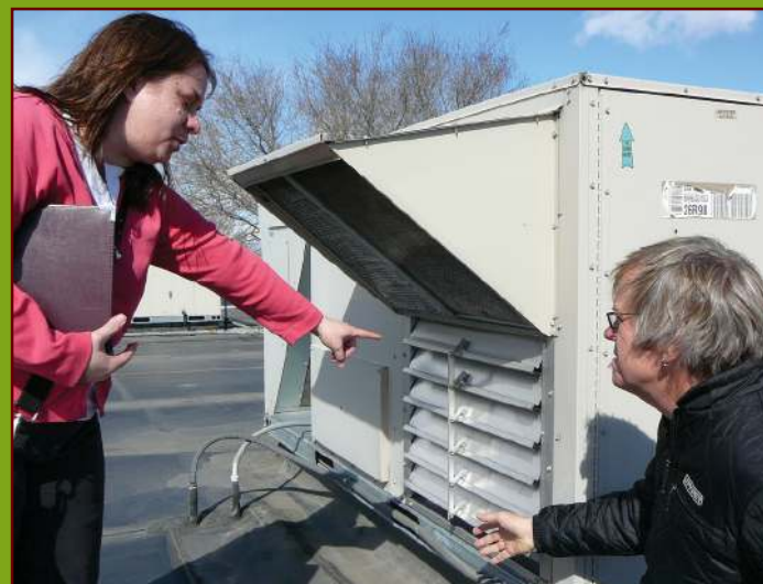
Climatewise helps their partners find ways to cut energy costs.
