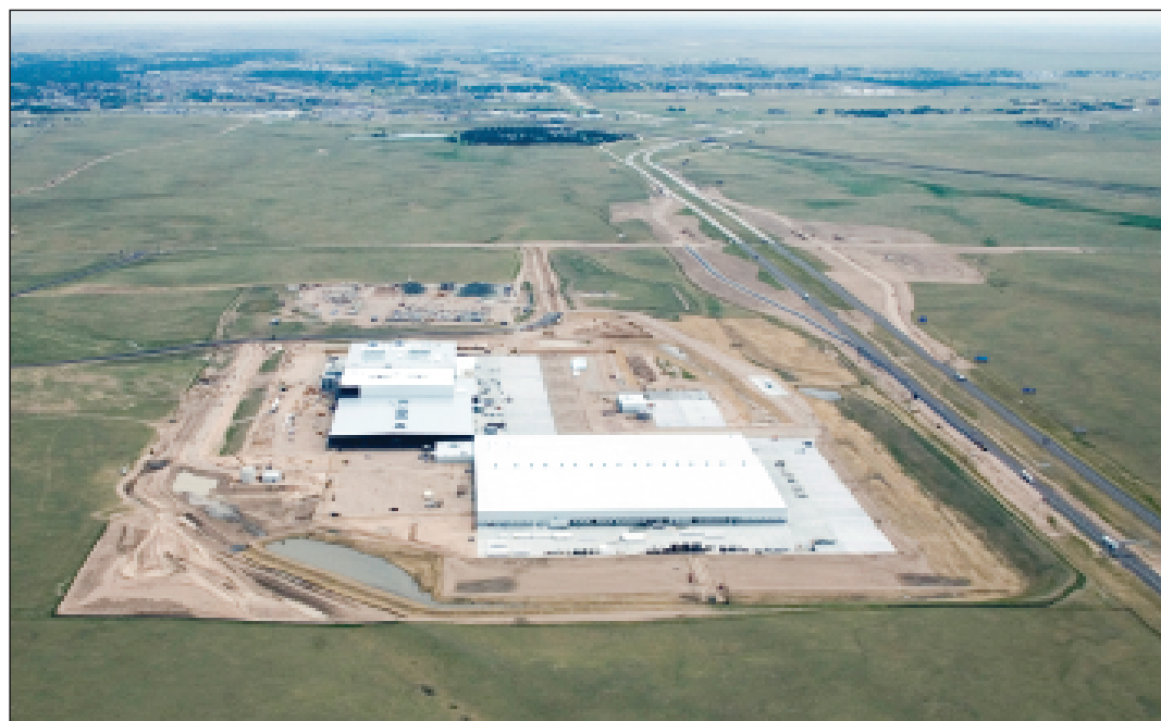
The 2005 announcement of Wal-Mart's Food Distribution Center to Cheyenne LEADS' North Range Business Park again highlighted the area on the economic development radar.
