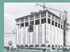
Mountain States Telephone and Telegraph Co. Colorado Springs Main Operating Building
