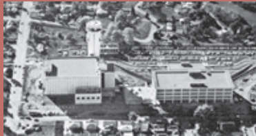
Mountain Bell Zuni Communications Center, Denver, CO
