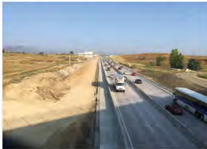
The construction project along U.S. 36 between Denver and Boulder is adding express lanes and improving interchanges along the busy corridor.
